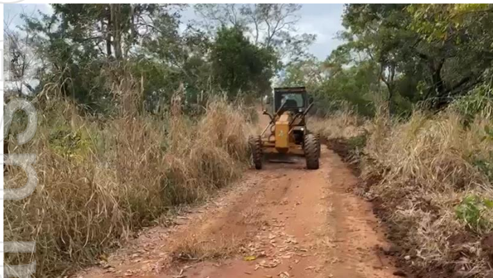
Grading of the Ancuabe main access road
