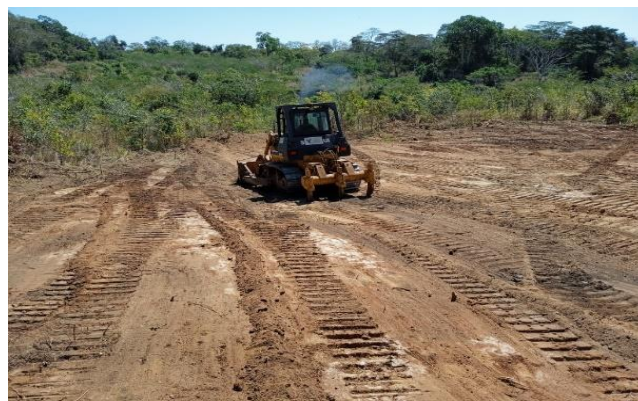
Clearing of regrowth at proposed water dam
